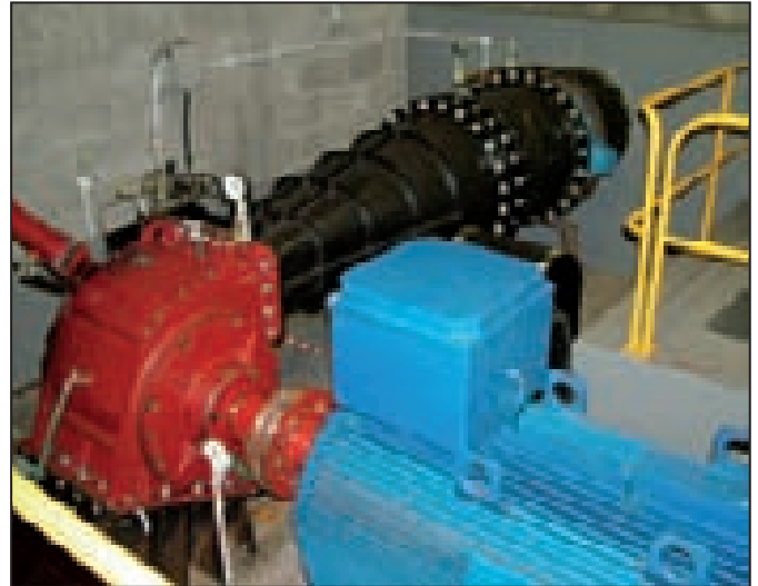
The turbine (shaft coupling has been removed for clarity)
