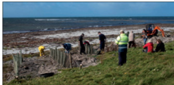
The second sand blow fencing completed
