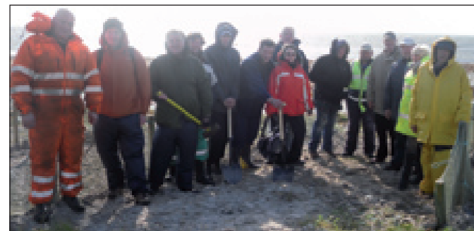
Community groups working to build the sand blow fencing
